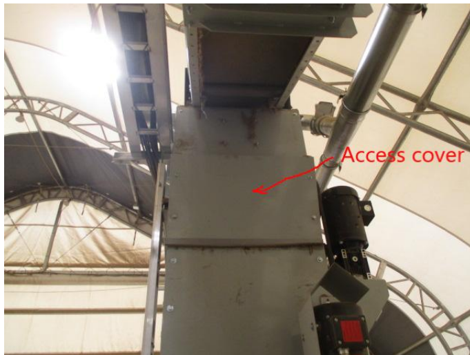
Figure 13 - Location of Primary separator access cover
