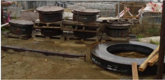
Autoclave Nozzles, Flanges (24")
